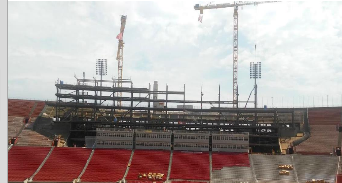
Los Angeles Memorial Coliseum Construction Site (Visited Week 5) PC: Soyoung Moon
